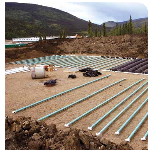
Constructing the Dispersion Field
