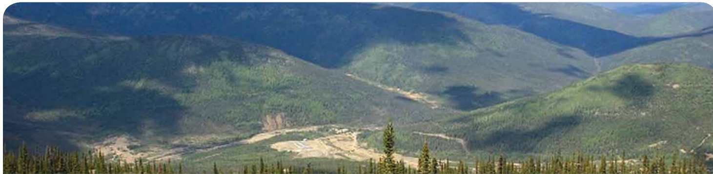
View of the location of the Eagle Gold Camp infrastructure from where the open pit will be situated.
