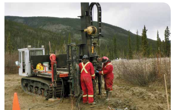
Geotechnical drilling where the Eagle Gold infrastructure will be located.
