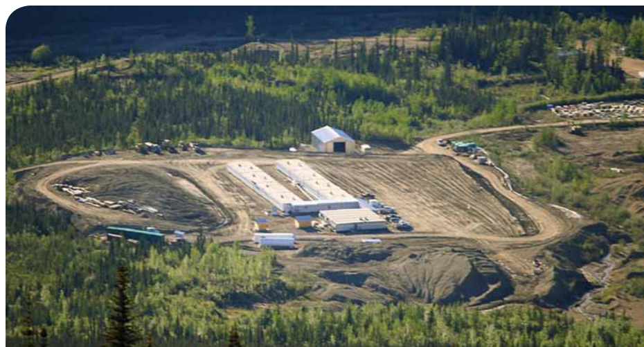
The new Dublin Gulch 100 person camp including the recently erected shop facility.
